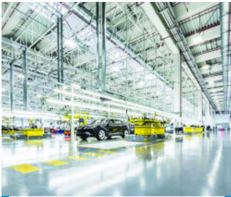
Fiber reinforced Concrete floor with Mapefibre ST 42
